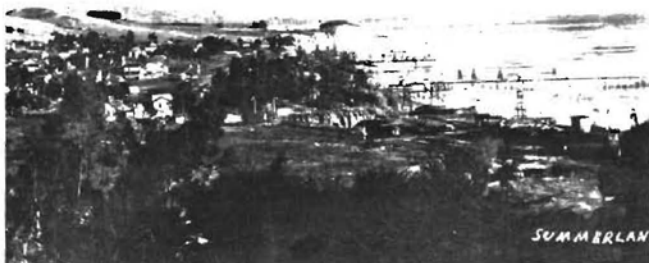
Summerland oil field, Santa Barbara County, around 1900. Onshore drilling started here in 1886. As field development continued, operators realized the oil sands extended under the ocean. To reach the offshore sands, piers were built over the water to support drilling and production machinery.
