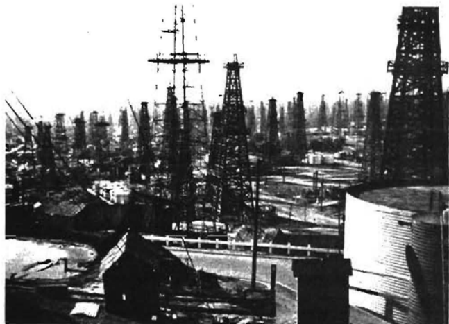
Signal Hill, a part of the Long Beach oil field, was a prolific oil producer. The Long Beach field reached its production peak of 68 million barrels in only 2 years after discovery.
