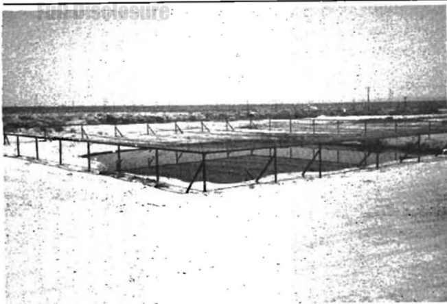
Screened oilfield sump in Southern California.
