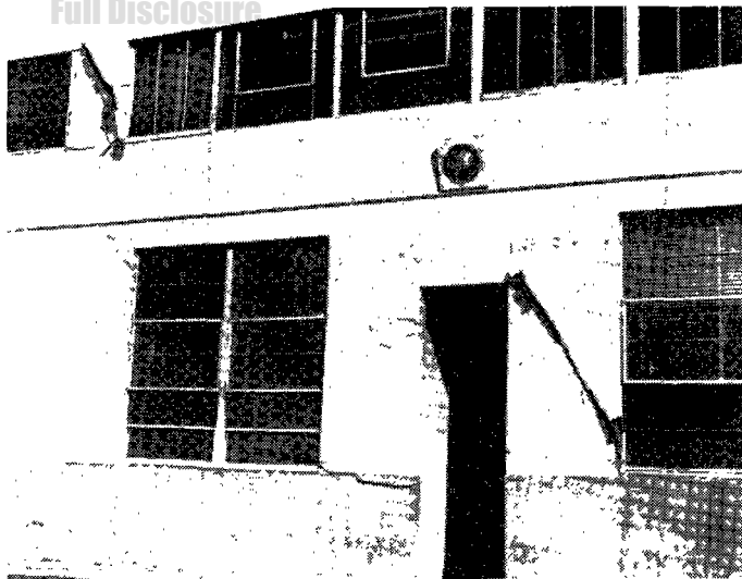
FIGURE 7. Shear Cracks on Wall
