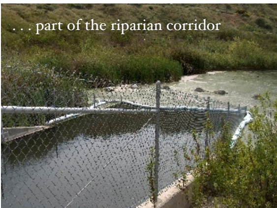
Playa Vista’s “wildlife crossing” under Lincoln Boulevard . . .
