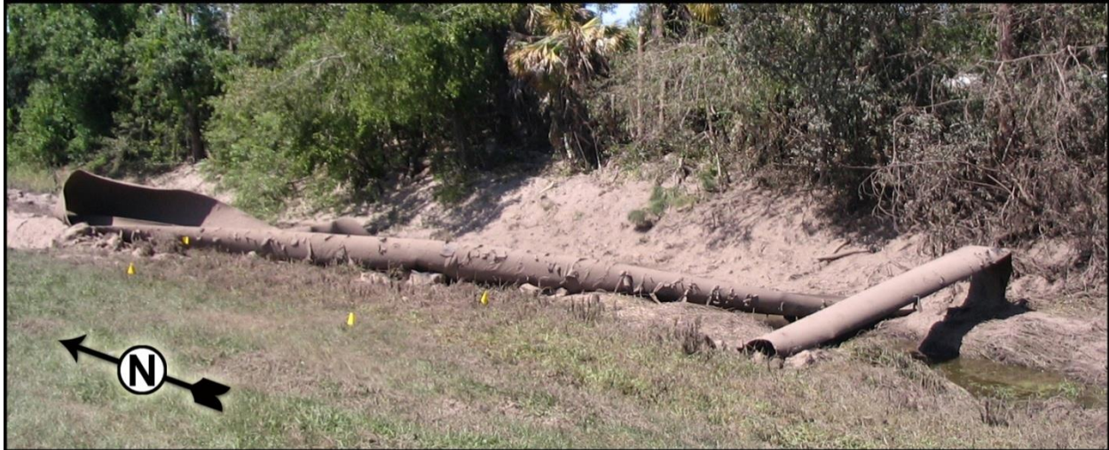
Figure 5. One hundred four-foot-long section of 18-inch buried pipe that was dislodged from the ground.
